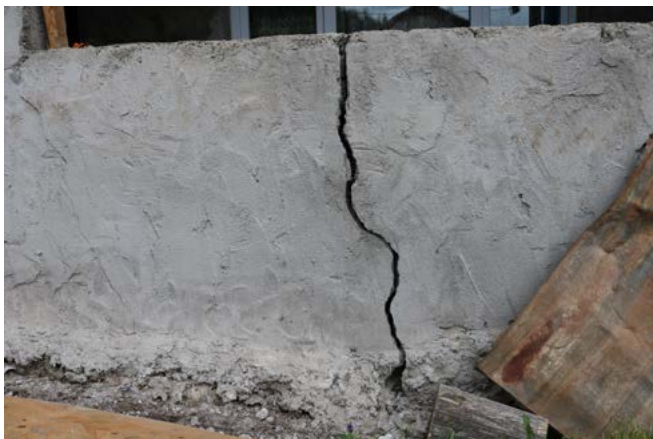
The wall of the Iakobadze family house cracked as a result of drilling and explosions of HPP construction, Ghurta village; "Shuakhevi - "Chronicle of HPP Foretold" 2019 © Green Alternative
