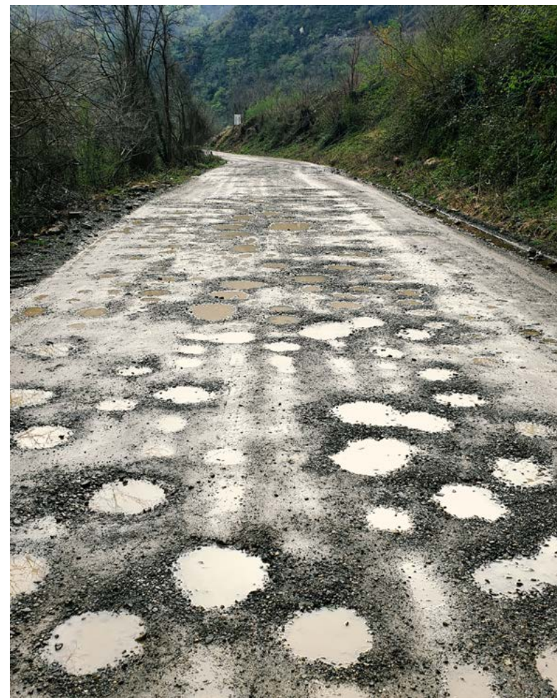
After the works of Namokhvani Cascade, the Kutaisi-Alpana-Mamisoni road was damaged by the heavy gear of “Enka” company.
